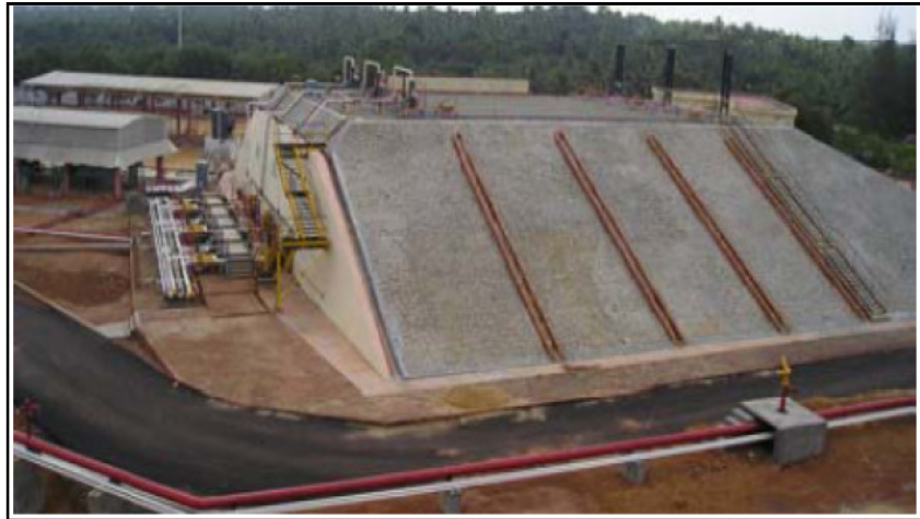
Figure 2. Mounded LPG Facility (Source:Fabtech)
